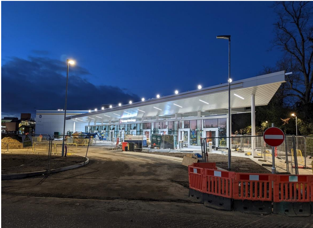
Stevenage Bus Interchange (Under Construction)
